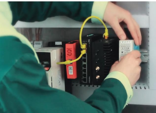
Installing TRENDnet's TI-PG80 industrial switch to the DIN-rail mount.
