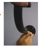
2. Drill holes for the fastener plugs at each marked position. Make sure the drill bit matches the size of the provided white screw anchors.
